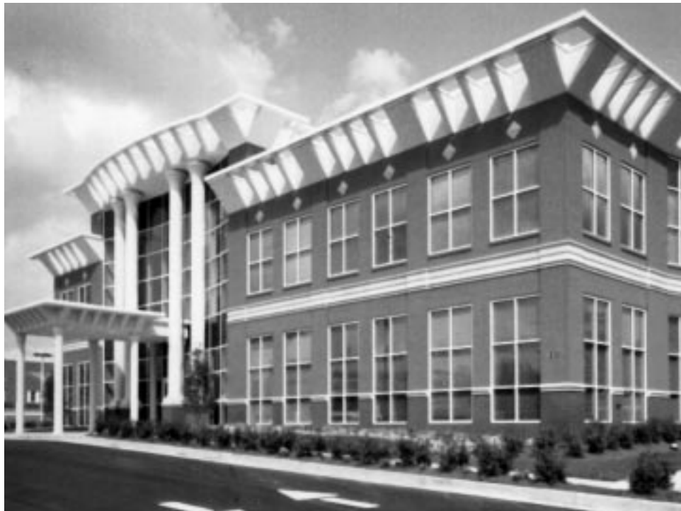
Regions’ Bank new facility.
